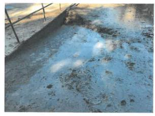
SOLIDS FILLED TO TOP.NO LONGEABLE TO DRAIN
